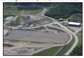
contractor began the closure project in 2019 and completed Stage 1 of the closure project in Fall 2020. The Stage 1 project consisted of soil stripping for stormwater protection, installing geotextile and geonet to existing landfill cover soil, infilling with an additional capping soil, installation of a geomembrane and finalizing the site work with topsoil and seeding.
