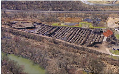
Green Waste Composting Facility
