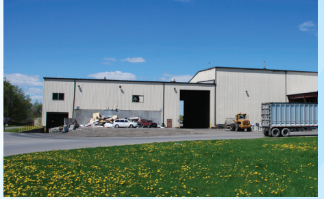
Three Solid Waste Transfer Stations
