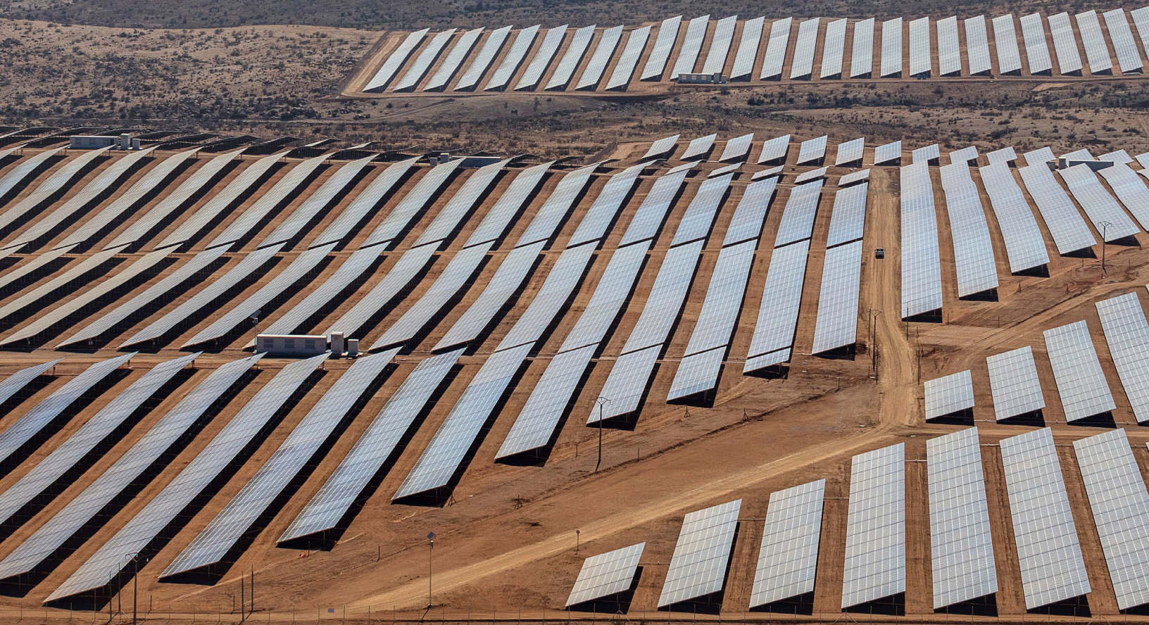
El Romero solar farm in Chile (80 MW for Google)
